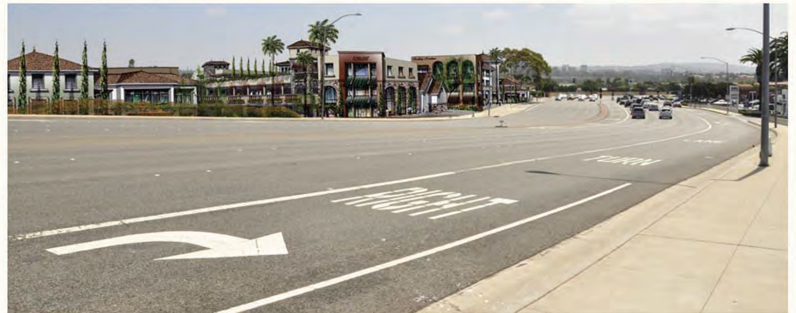
View from Bridge along East Coast Highway
